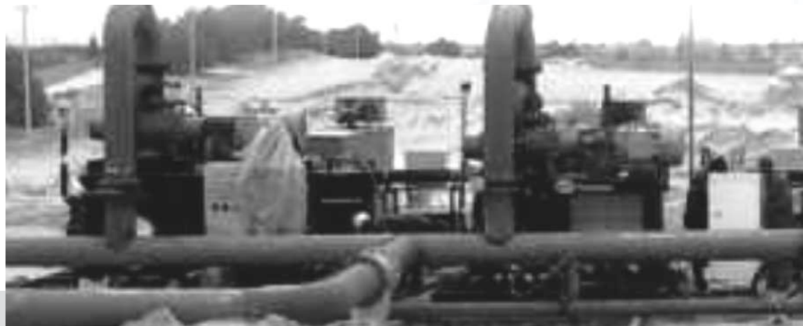
Vacuum Drying of Gas Pipe Lines
